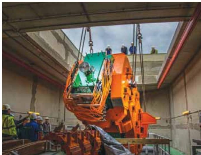
*The MedAustron MBV-F magnet being lowered into Irradiation Room 2. (MedAustron)*
